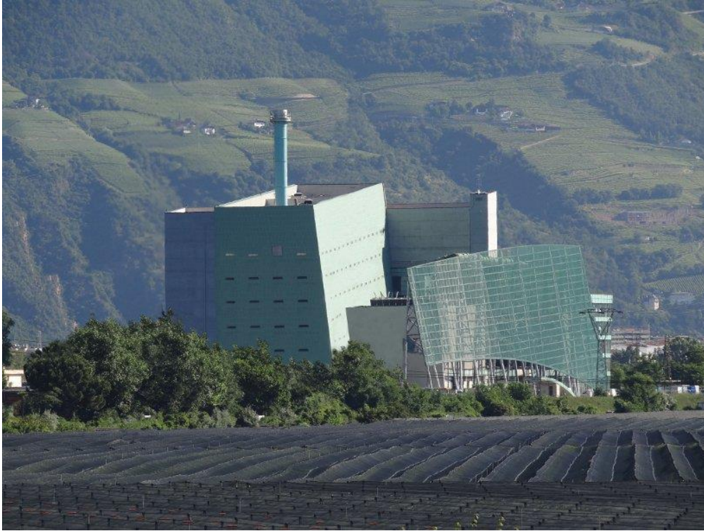
Fig. 39. Waste incineration plant in Bolzano.
