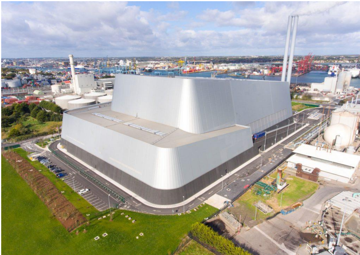
Fig. 28. Dublin waste incineration plant.
