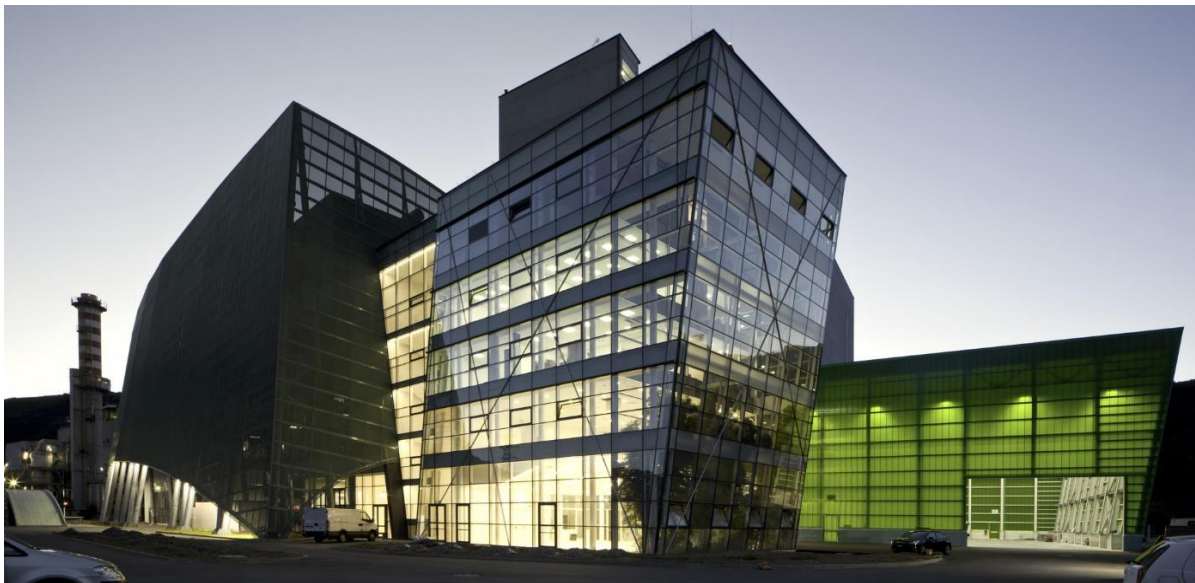
Fig. 35. Waste incineration plant in Bolzano.
