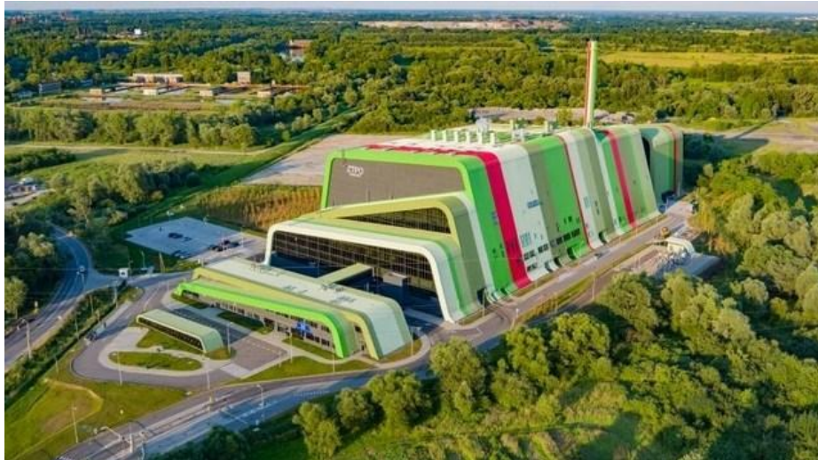
Fig. 21. Waste incineration plant in Krakow.
