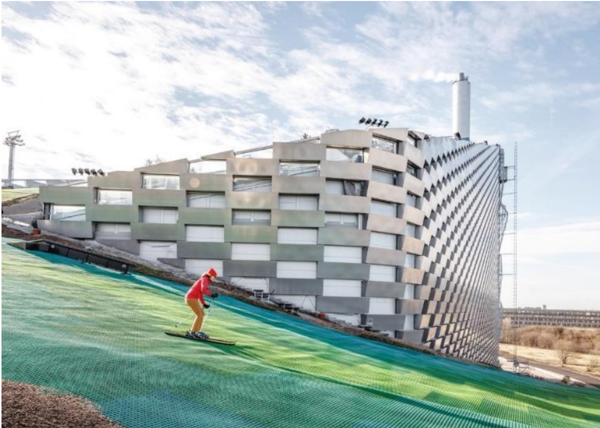
Fig. 14. “Copenhill” – waste to energy plant in Copenhagen.
