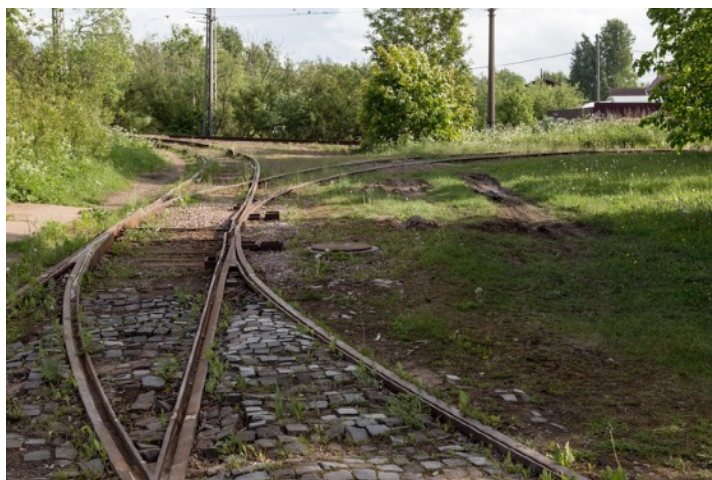
Oranela tram rails nowadays
