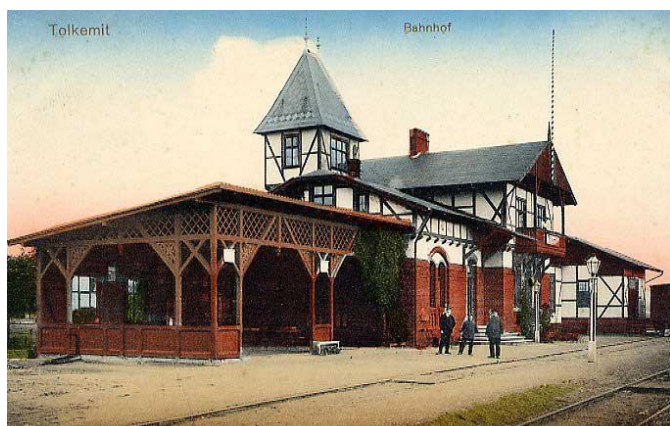
Photo 5. Tolkemicko railroad station around 1900 Source: wolneforumgdansk.pl
